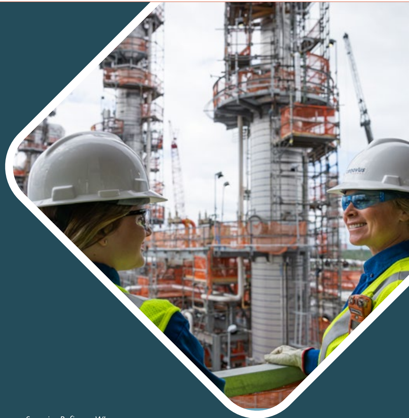
▲ Superior Refinery, WI
