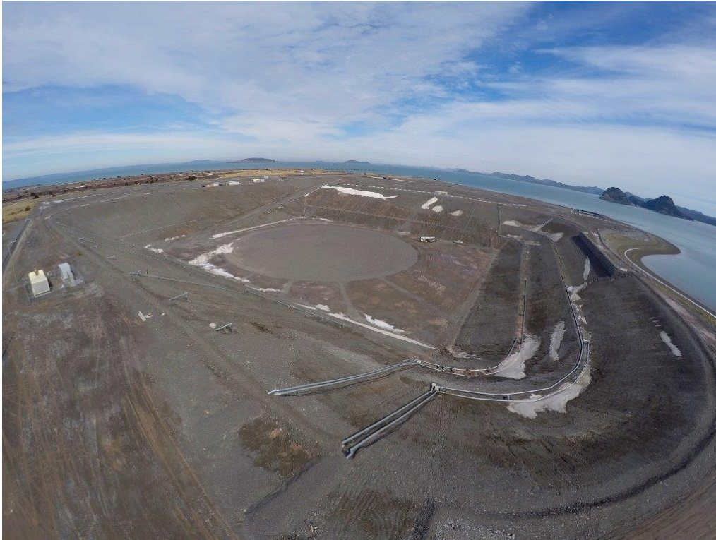
Completed Graving Dock at Argientia
