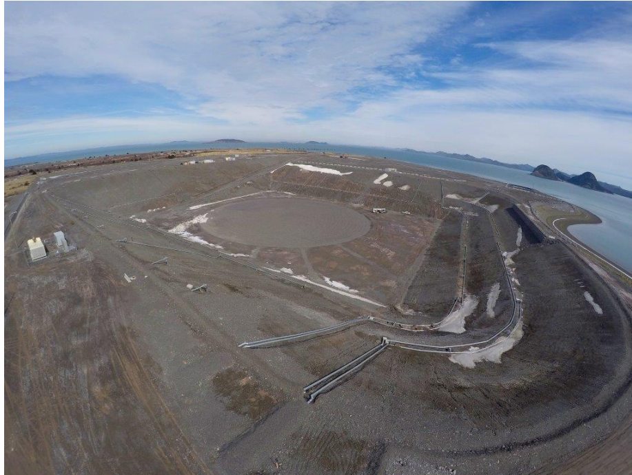
Completed Graving Dock at Argentina
