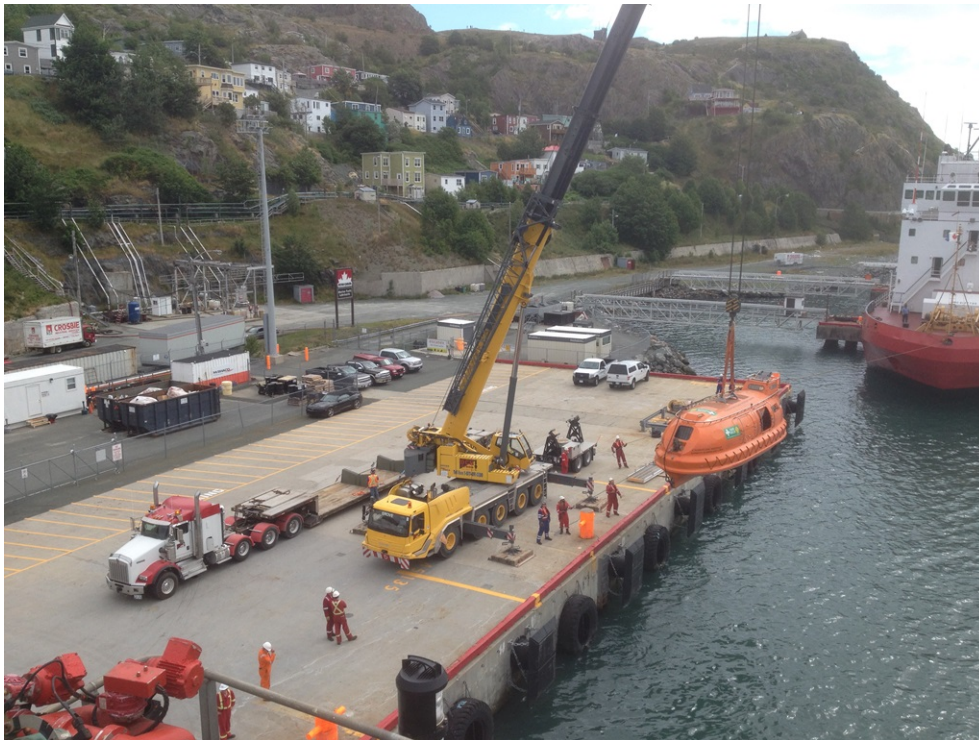
Preparation for Fit Testing of Wellservicer Lifeboat to SeaForce HRF
