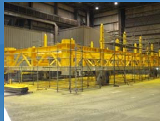
MSF #2 – partially painted
